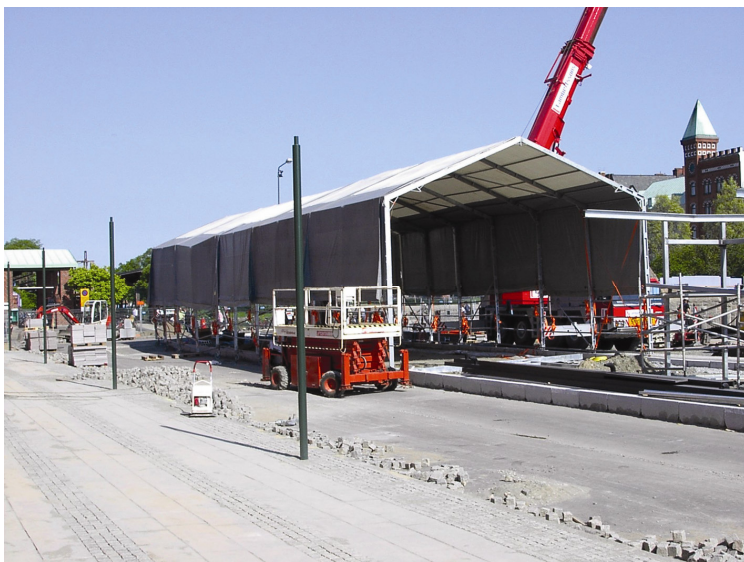
Figure 6.1 Commonly utilised type of weather protecting tent (Jonsereds, 2002).
