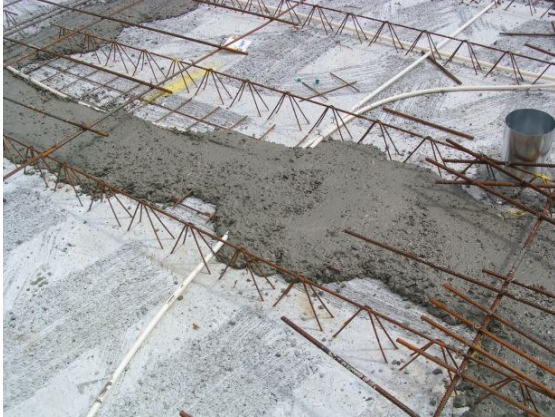
Figure 4.9 In order to avoid leach of high flowable SCC between formwork joints, the first concrete delivery for each slab casting consisted of SCC with reduced slump flow, which was placed by moving the pump mast over the interfaces.
