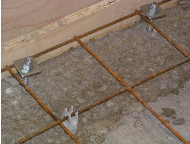
Figure 5.13 The second specimen incorporated reinforcement net, anchored to the HD/F-elements.
