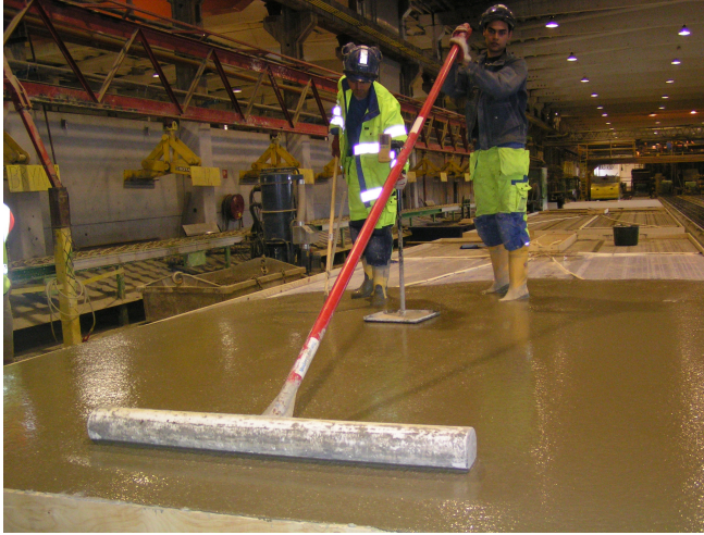
Figure 5.7 SCC full-scale casting simulating 'real' conditions.
